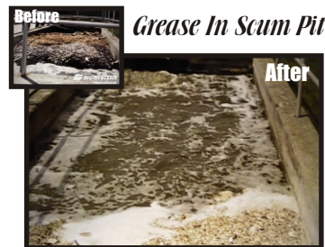
Grease in a Scum Pit:
